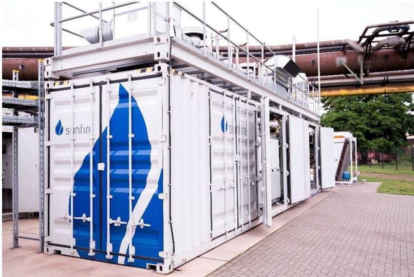
GrInHy2.0 high-temperature electrolyzer at Salzgitter's steel works (© Salzgitter AG)
